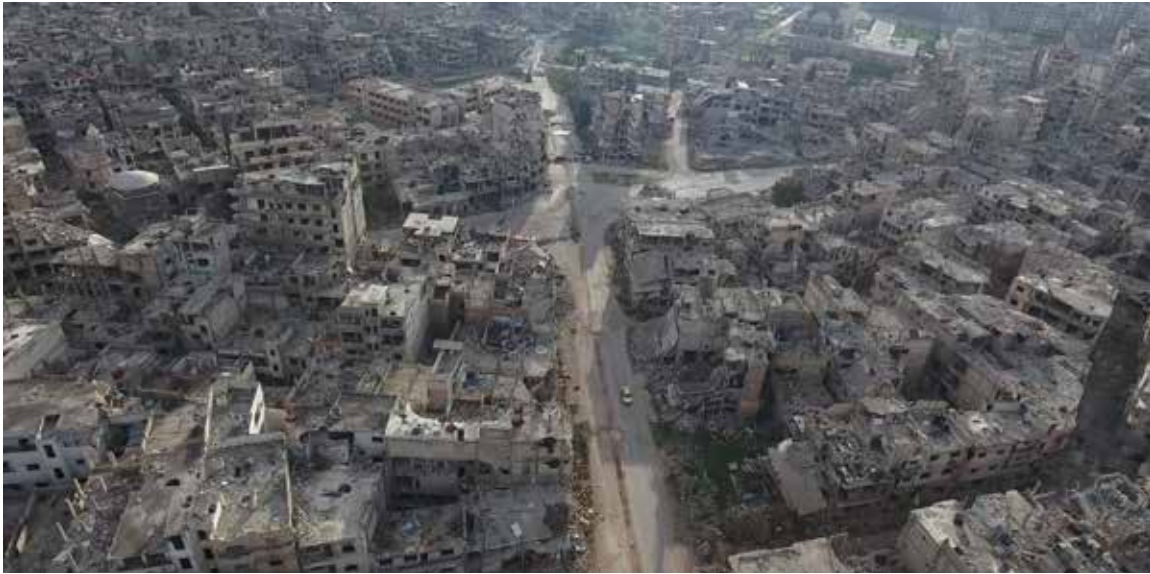
Shelling and air strikes left the dense urban areas of Homs in ruins. Source: Karam Almasri / Shutterstock
