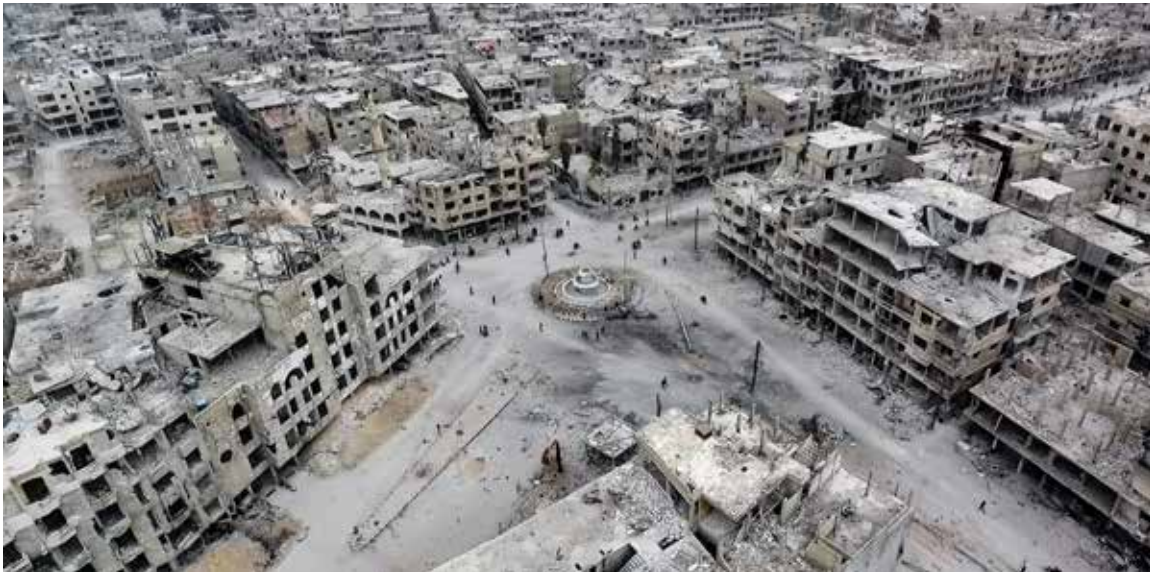
Wreckages of structures of Arbin town in Eastern Ghouta, which has been under siege by the Government of Syria, March 27, 2018. Photo by Ammar Al Bushy/Anadolu Agency/Getty Images
